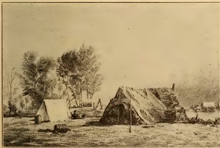
ELKHORN RIVER CROSSING
